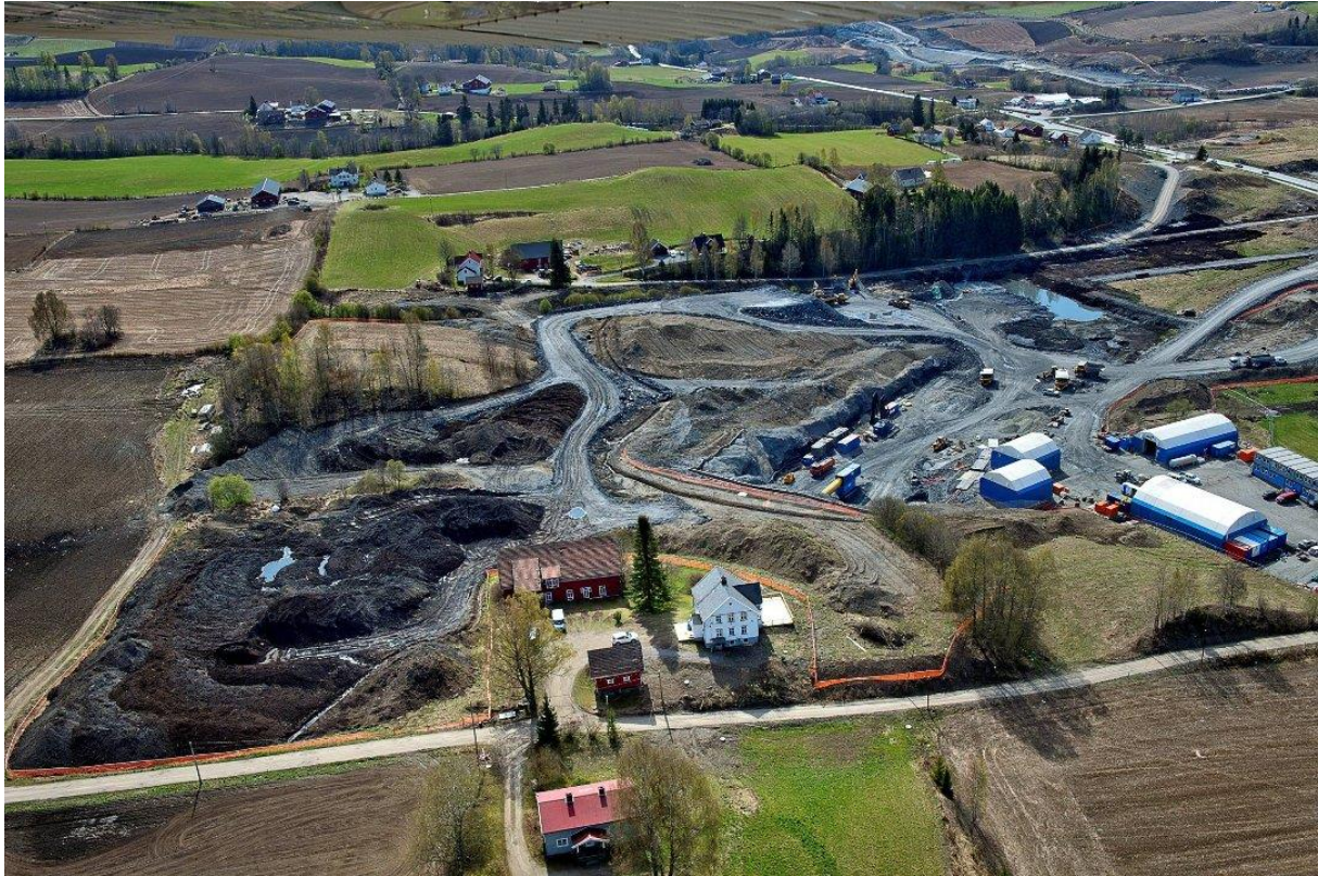
Figure 5: Aerial photo (Eidstuen, 2014) of the area around the Southern tunnel opening at Rv. 4 Gran, underneath Morstad farm in front. The alum shale depot is located to the upper right of the photo.
